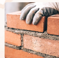
READY TO CONSTRUCT
